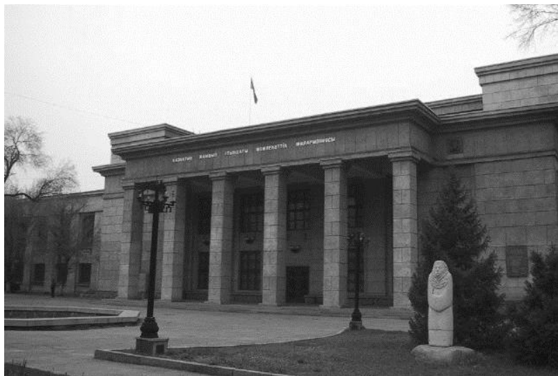
Fig.2: The building of CUFS – now the Central Concert Hall of Almaty Philharmony
